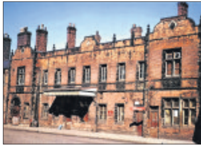
South Staffordshire Railway Station building, about 1965
